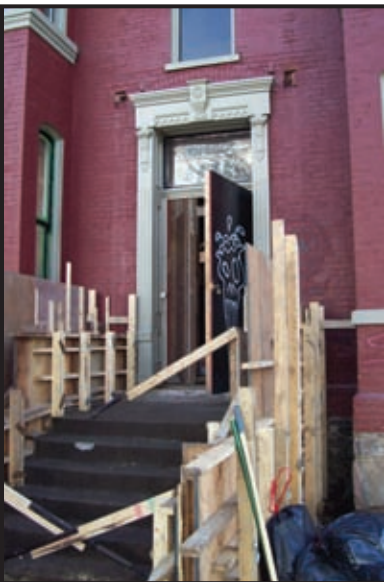
front porch rebuilt
