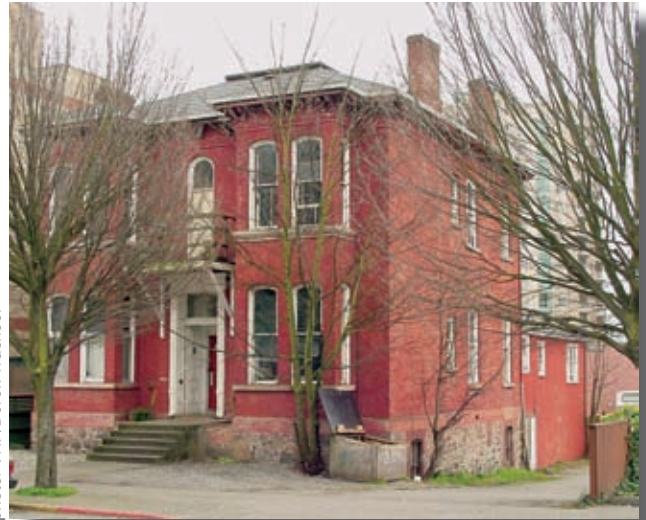
1007 Johnson in 2002, missing front porch & widow's walk
