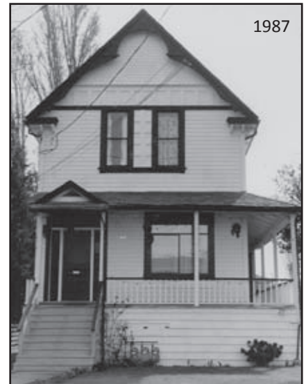
Many wood windows were replaced with aluminum, including the front Queen Anne window. Gable ornament lost.
